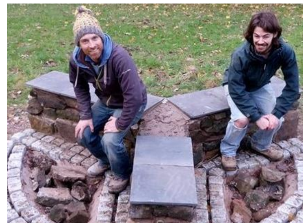
Volunteers Peter Whittle & Ben Cooper at the new seating area in Scotch Quarry
